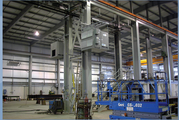
UAS Smog-Hog systems are arranged in a racetrack configuration.
